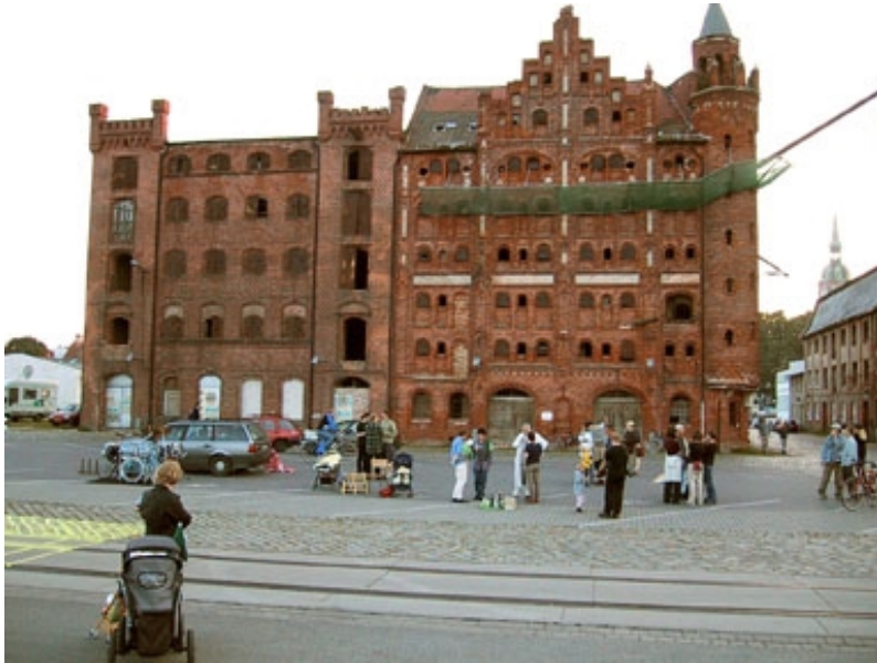
speicher 9/10 seen from waterside
